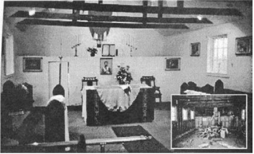
The Chapel of Christ the King, at St Gregory's Retreat Center and Farm, before (inset) and after. Many hands and talents went into working this transformation.
